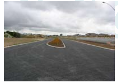
New traffic lanes on Wairere Drive.
