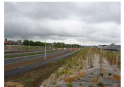
Planting on the noise bunds.
