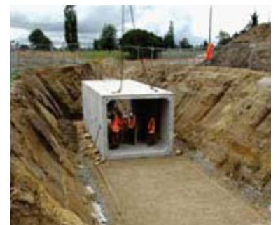
Underpass installation at the new roundabout intersection.
