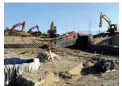
Construction of roundabout internal retaining walls.
