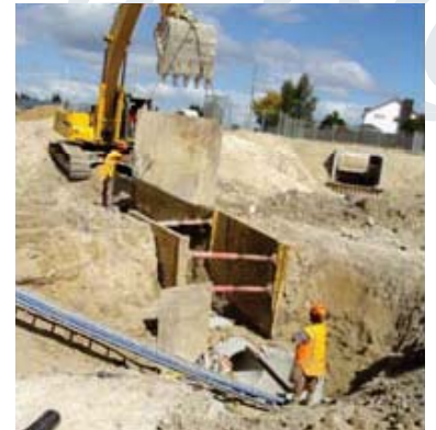
Installation of stormwater connections under the new roundabout.
